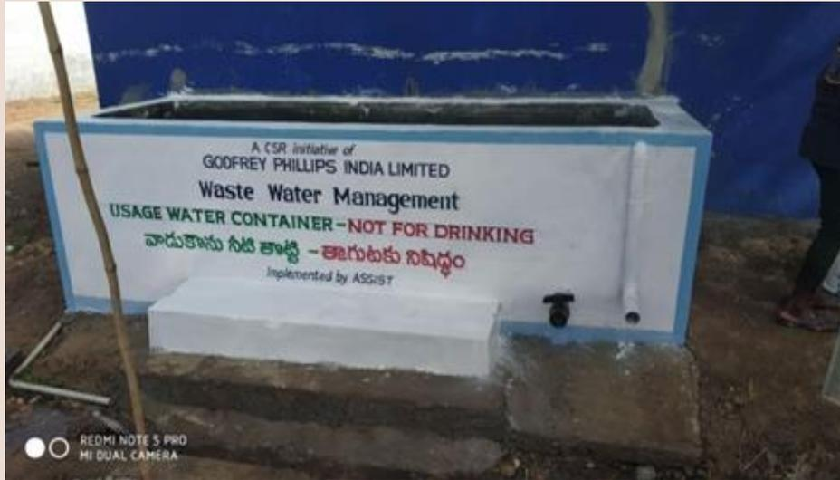
The RO plant while providing safe drinking water also wastes upto 75%. The water with the impurities may leach into the ground. To avoid that the Community RO plants are being fitted with tanks or recharge pits like borewell to keep the ground water intact.
